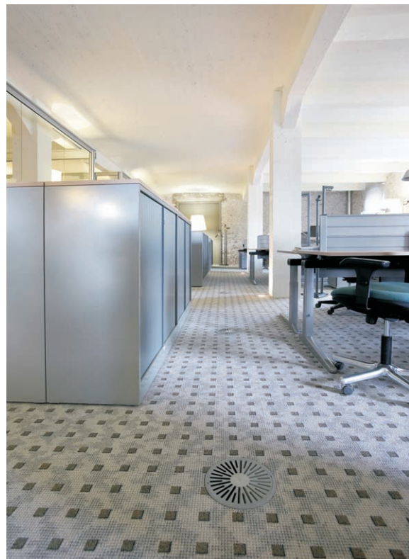
Figure 6: Floor twist outlet in an office
